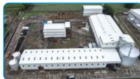
300 TPD Solvent Plant Boiler Capacity : 6 TPH 17.5 Kg
