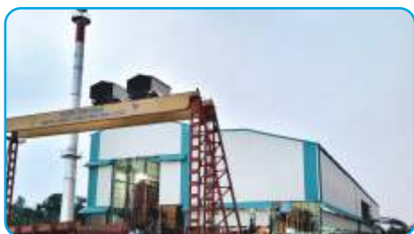
1000 TCD Boiler Capacity - 20 TPH 45 Kg 410 0 C Power Turbine : 2 Mw
