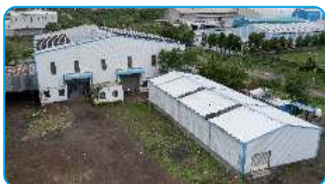
60 TPD Hygienic Dal Mill Pulses UnLoading to Product Bagging Colour Sortex, Magnetic Separators
