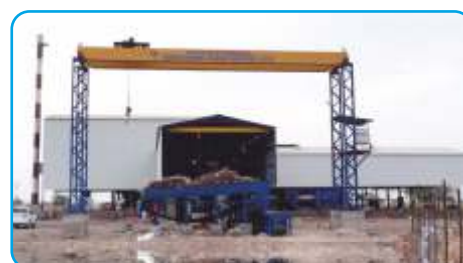
200 TCD Boiler Capacity : 6 TPH 32 Kg 380 0 C Power Turbine : 250 Kw
