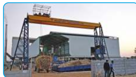
600 TCD Boiler Capacity : 10 TPH 32 Kg 380 0 C Power Turbine : 1 Mw
