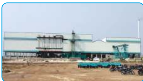
700 TCD Boiler Capacity : 15 TPH 32 Kg 380 0 C Power Turbine : 1 Mw
