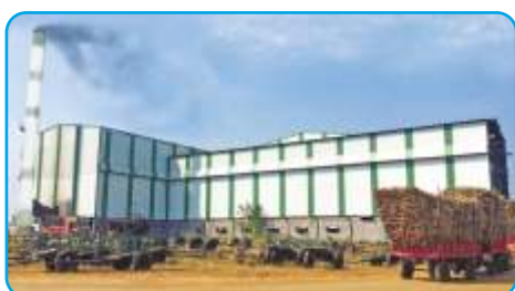
1000 TCD Boiler: 25 TPH 45 Kg 380 0 C Turbine : 2 Mw
