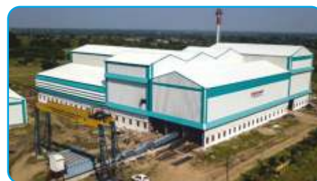
700 TCD Boiler Capacity - 15 TPH 45 Kg 410 0 C Power Turbine : 1.5 Mw
