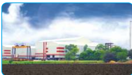
1400 TCD Boiler Capacity - 25 TPH 45 Kg 410 0 C Turbine : 2 Mw
